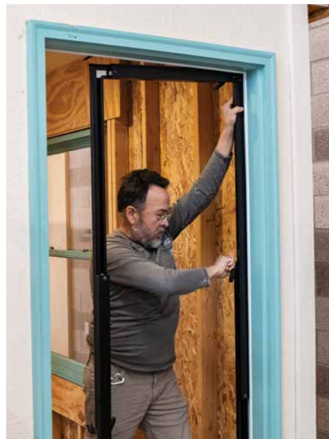
Left: Instructor Gerardo López and a student perform combustion analysis on a water heater; Above: López sets up a blower door in the ESA lab and performs a blower door test
