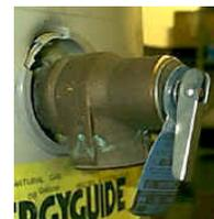
machine is “low” or “high” temperature. A TPR valve is also present on the booster heater supplying hot sanitizing rinse water to “high temp” machines. TPR valves have a limited service life and will eventually fail.
